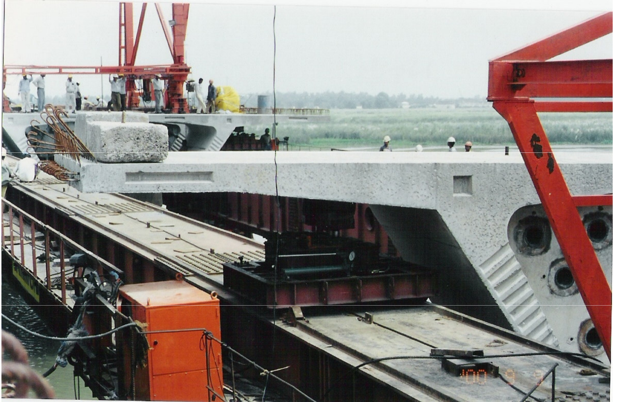
SUPPORTING TROLLEY FOR THE SEGMENT TO MOVE OVER
